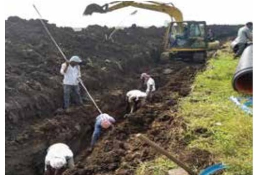
As mentioned in IS: 16098 (Part-2), excavated soil shall not be deposited near trench. This is in order to prevent the collapse of the sides of trenches. The sides of trench shall be supported by shoring, if necessary, to ensure proper excavation and to reduce the time of excavation. If excavation is made deeper than necessary the soil shall be backfilled and compacted.
